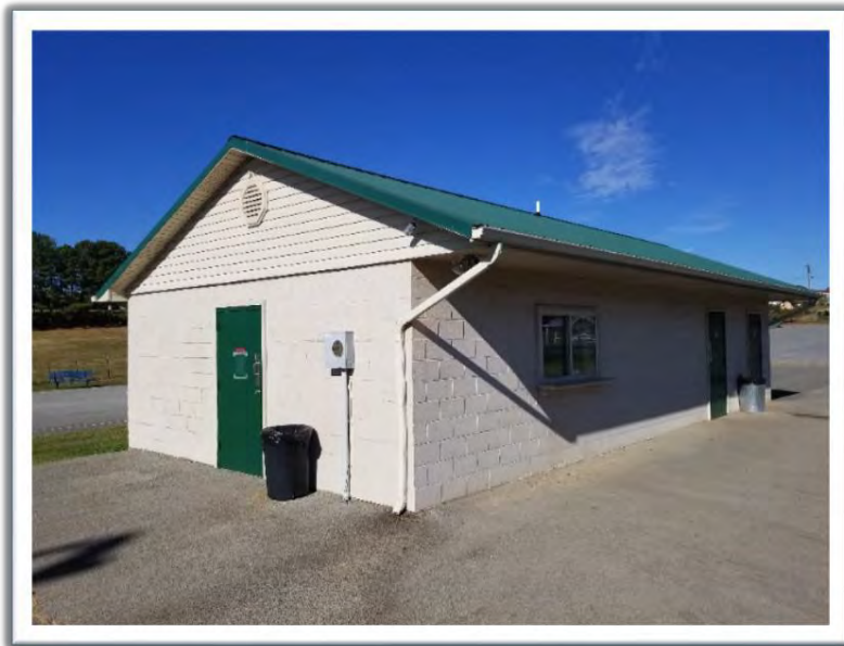
Concession and Restroom Building
